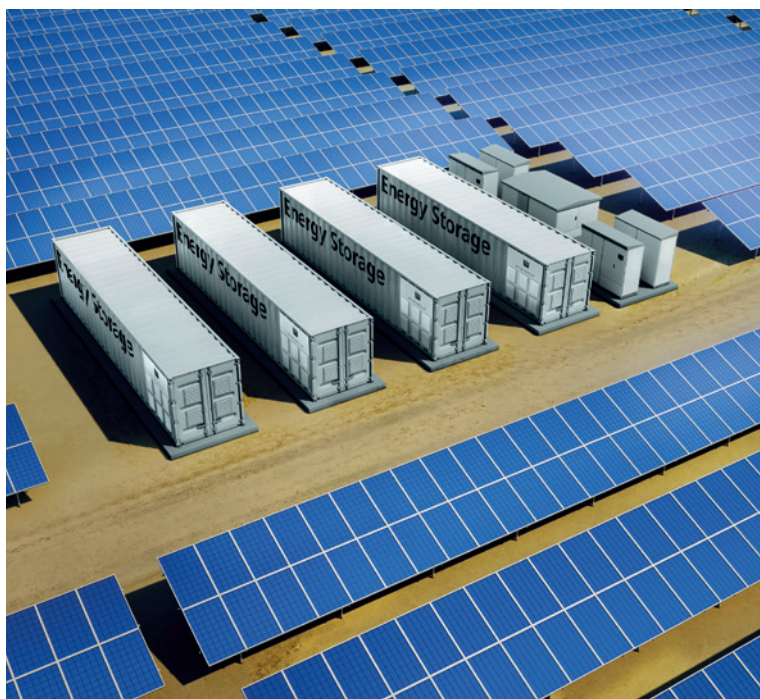
An artist's impression of a 2 MW/12 MWh single PV-Battery block
